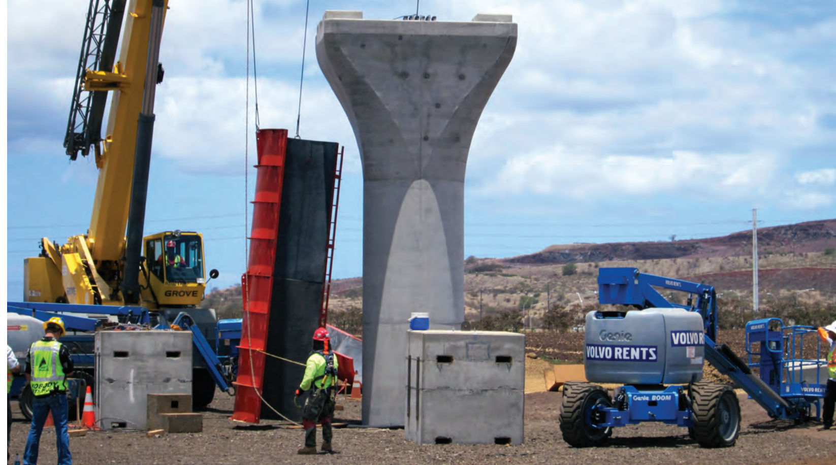
A construction crew removes the casting mold from the first support column for the Honolulu rail transit system
